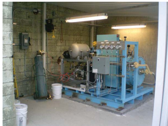
FIGURE 4. The custom 50 \text{ m}^3/\text{hr} compressor for the JENSA gas jet target as installed at the HRIBF.
