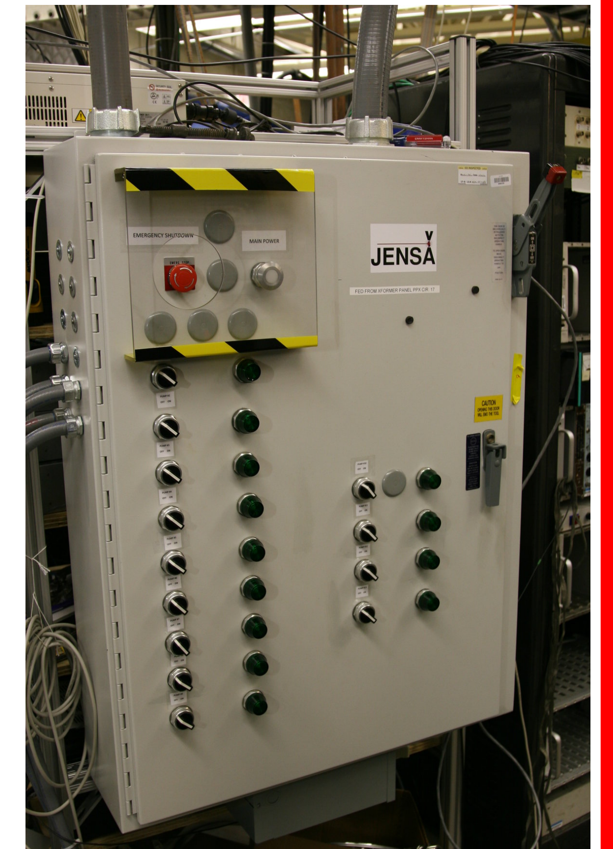
Above: Control panel for the JENSA system roots blowers
